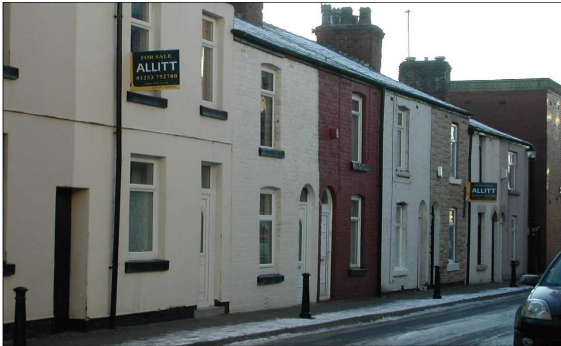
Caroline Street – Typical workers housing
