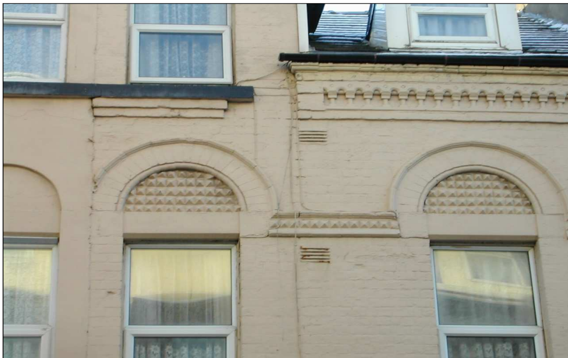
Terracotta details, now painted, Bairstow Street
